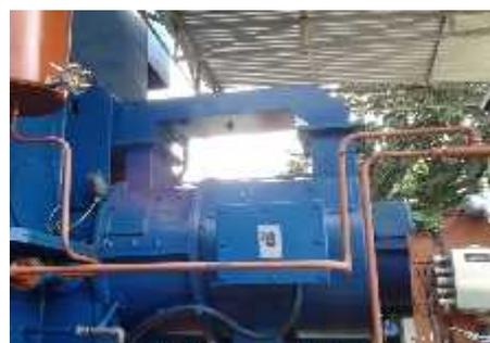
Gambar 4 Exciter Generator Gas Unit LM2000 PLTG Borang
