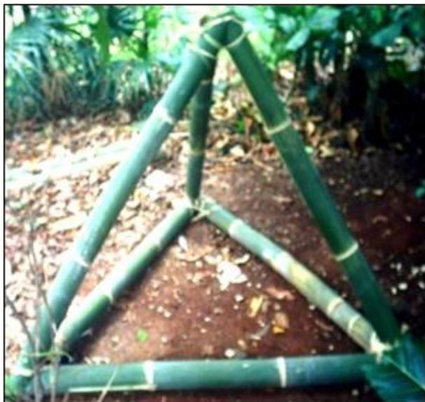
**Gambar 2. Terumbu Buatan Bambu**
