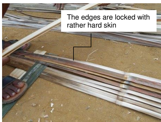
Figure 5. The process of weaving bamboo walls.
