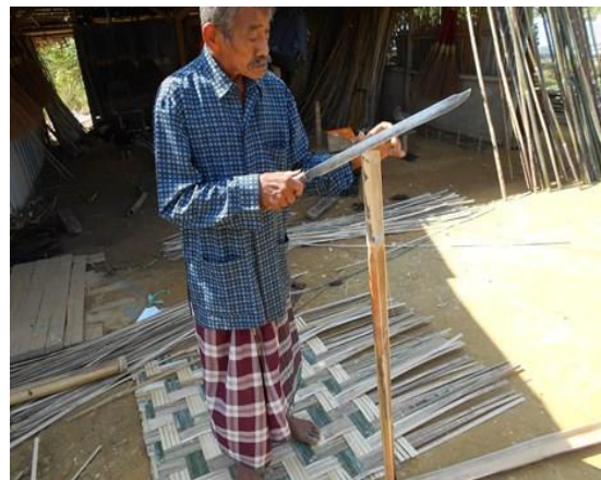
Figure 1. Making bamboo walls
