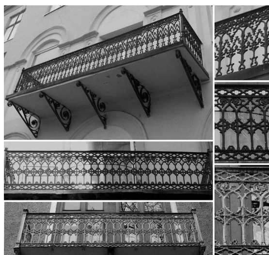
Fig. 4. Cast balcony fencing on the buildings situated at: 29, Halytska Str. (dated 1835); 2, Bachynsky Str. (dated 1874–1880); 4, Shevchenko Str. (dated 1880th)
