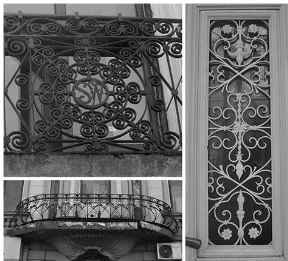
Fig. 6. Balcony fencing on the house № 26 at Sichovyh Striltsiv Str. (dated 1894); on the building № 12 at Market Square (1880); metal-plastic of door panel on the house № 104 at Shevchenko Str. (1896)
