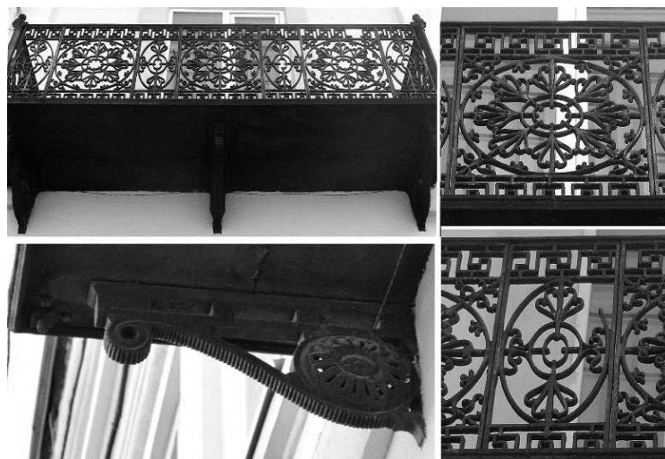
Fig. 2. Balcony fencing and balcony bracket on the building number 2 at Starozamkova Street (1732)
