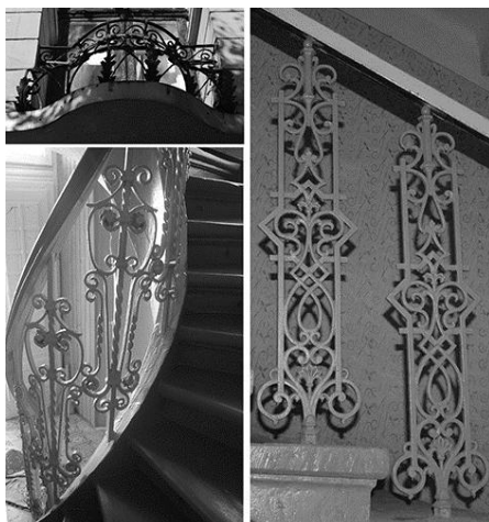
Fig. 7. Balcony fencing situated on the house № 10 at Mazepa Str. (1896), staircase fencing in the building № 102 at Shevchenko Str. (1896–1897) and in the building № 11 at Mazepa Str. (1890)
