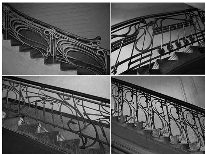
Fig. 8. Staircase fencing in the building № 26 at Chornovil Str. (1906); house № 5 at Vasylianky Str. (1911); house № 3 at Garkusha Str. (1912); building № 1 at Hrushevsky Str. (1910)
