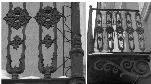
Fig. 3. Cast balcony fencing and brackets on the building situated at 1, Mazepa Str. – Vichevyi Square (dated 1827–1830)
