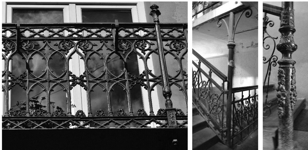
Fig. 5. Balcony fencing and brackets; staircase fencing; fragment of the decoration of staircase footing in the house №6 at Mazepa Str. (dated 1885)
