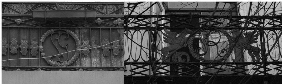
Fig. 1. Balcony fencing on the buildings situated at: 1, Mazepa Str. – Vichevyi Square (1827–1830); 18, Sichovyh Striltsiv Str. (1827)
