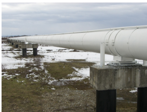
Fig. 1. Aerial “Urengoy-Pomary-Uzhgorod” gas pipeline crossing above Bystrytsia Solotvynska River (Ukraine)
