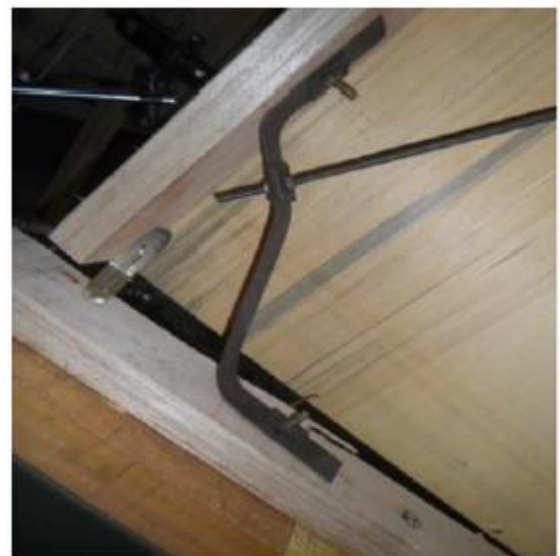
(c) Nail Pull-Through of Sheathing
