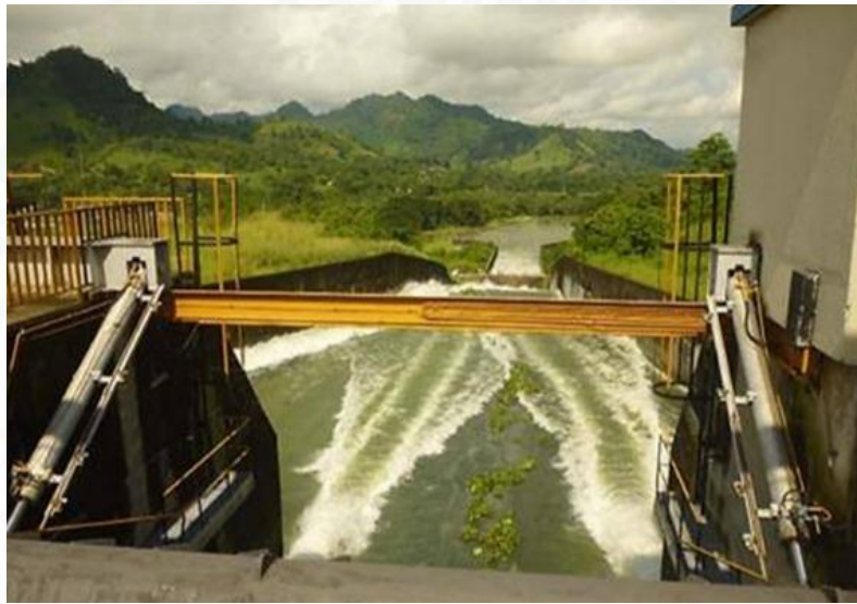
Figure 2. Gate of the La Esperanza Dam
