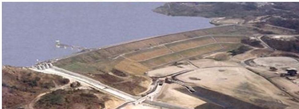
Figure 1. Image of the La Esperanza dam
