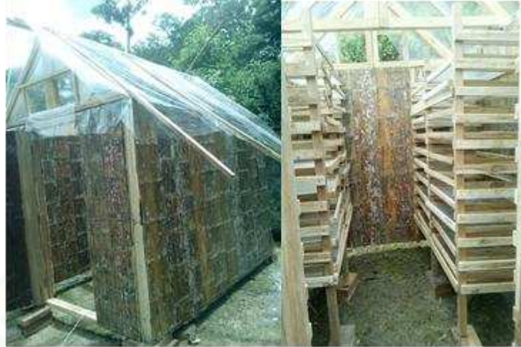
Figure 4. Solar grain dryer built with cane Guadua
