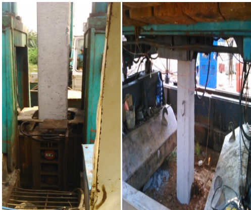
Gambar 8. Clamping & Piling
