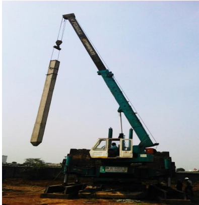
Gambar 7. Lifting pile
