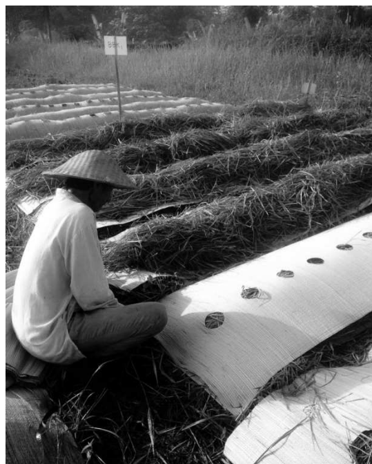
Figure 1. Biogeotextile installation
