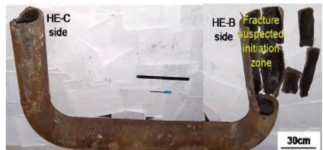
Fig. 1. General view of the fractured U-bend pipe joint connecting the heat exchanger B (HE-B) to the heat exchanger C (HE-C).
