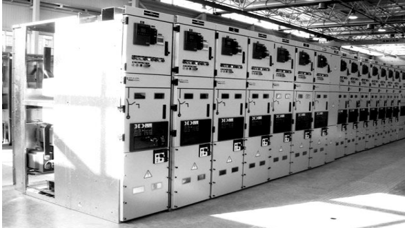
Fig. 2. 20 kV metal-clad switchgear (indoor switchgear equipment). [3].
