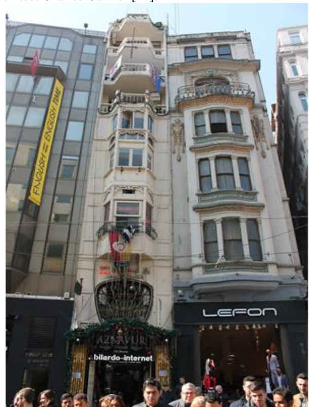
Figure 7: The façade of Aznavur passage in Istanbul.
