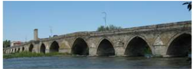
Figure 7: The Old Bridge.
