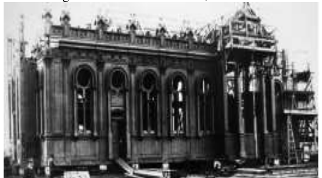
Figure 18: Construction phase of the church—iron structure
