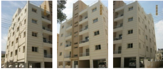
Figure 3. From right to left. North, South and East façade of the Uzun apartment 10 (research's field study, taken by author, 2016).
