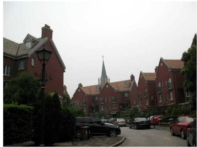
Figure 24. Shanghai Thames Town residential quarters in the Songjiang County imitating the Olde England. Photo: Donia Zhang 2014.
