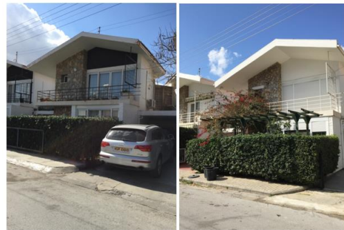
Figure 17. Exposed stone facades in Efruz Houses.
