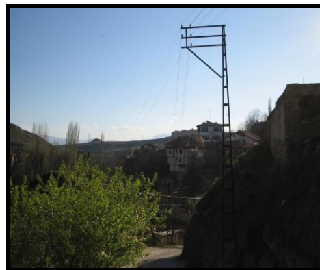
Figure 7 One of the electric poles in the city.
