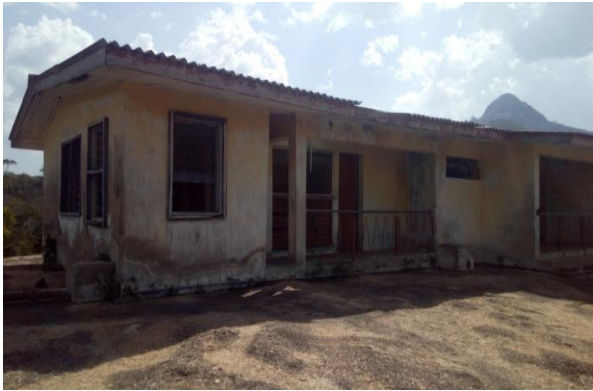
Figure 3: Guest/Tourist Chalet in poor condition, Oke Idanre.
