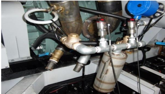
Fig. 4 Photo of Measuring Condition ②
