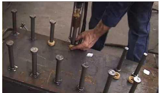
Figure 1. Shear connector
