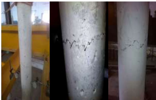
Fig 14: Showing Failure of Conventional Steel, 50%GFRP with GGBS And 100% GFRP Long Column and Central Crack Before Failure
