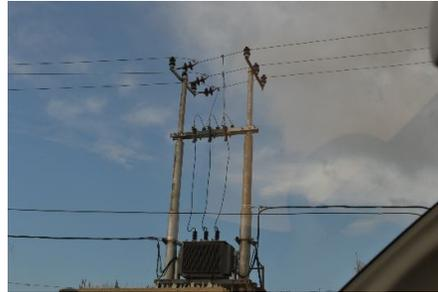
Gambar 1. Transformator 100 kVA
