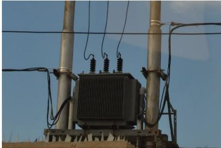
**Gambar 3. Transformator Distribusi Rufe Pantai 100 kVA**
