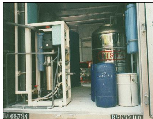
Gambar 14 : Pengolahan Air Sistem Reverse Osmosis Mobile Unit 10 m 3 /hari.
