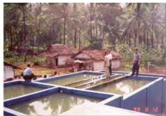
Figure 8. An example of slow sand filter of water purification reactor.
