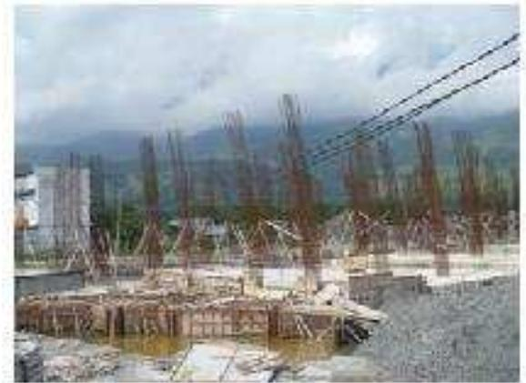
**Gambar 8.** Pengecoran lean concrete
