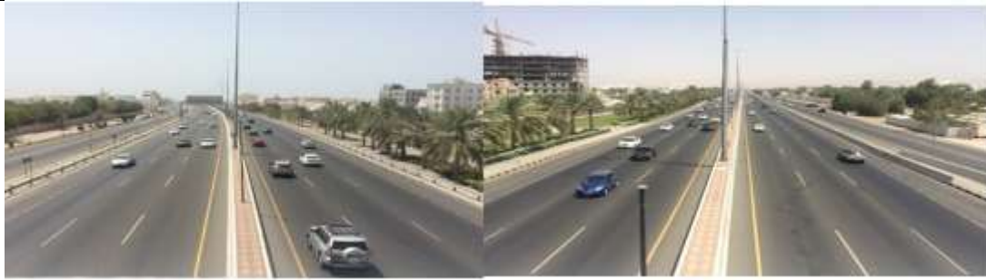
Fig. 7: Road Segment selected for implementation of the Smart Road Technology
