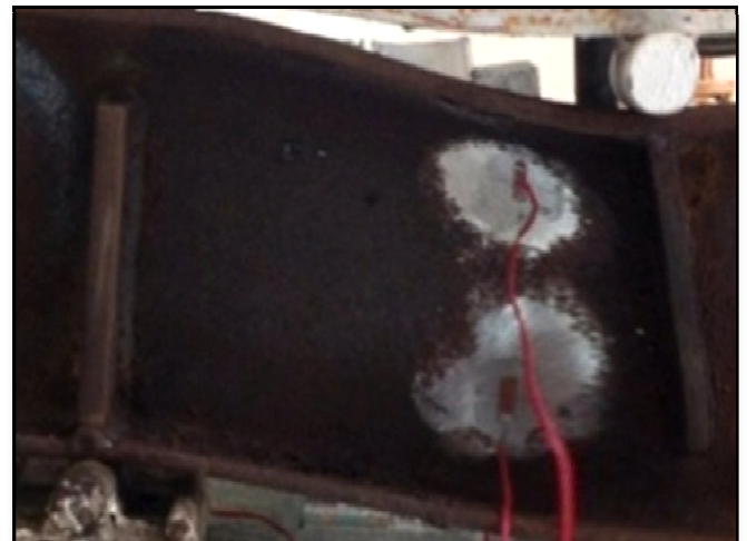
Figure 9: Failure due to web crippling.
