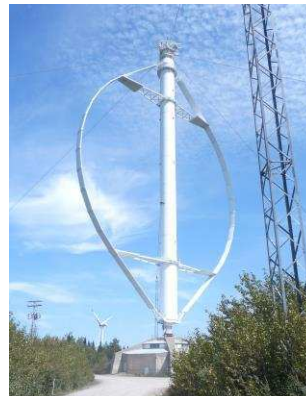
Fig. 4: Vertical-axis wind turbine – Darrieus-type. Source: Wikipedia, 2018.
