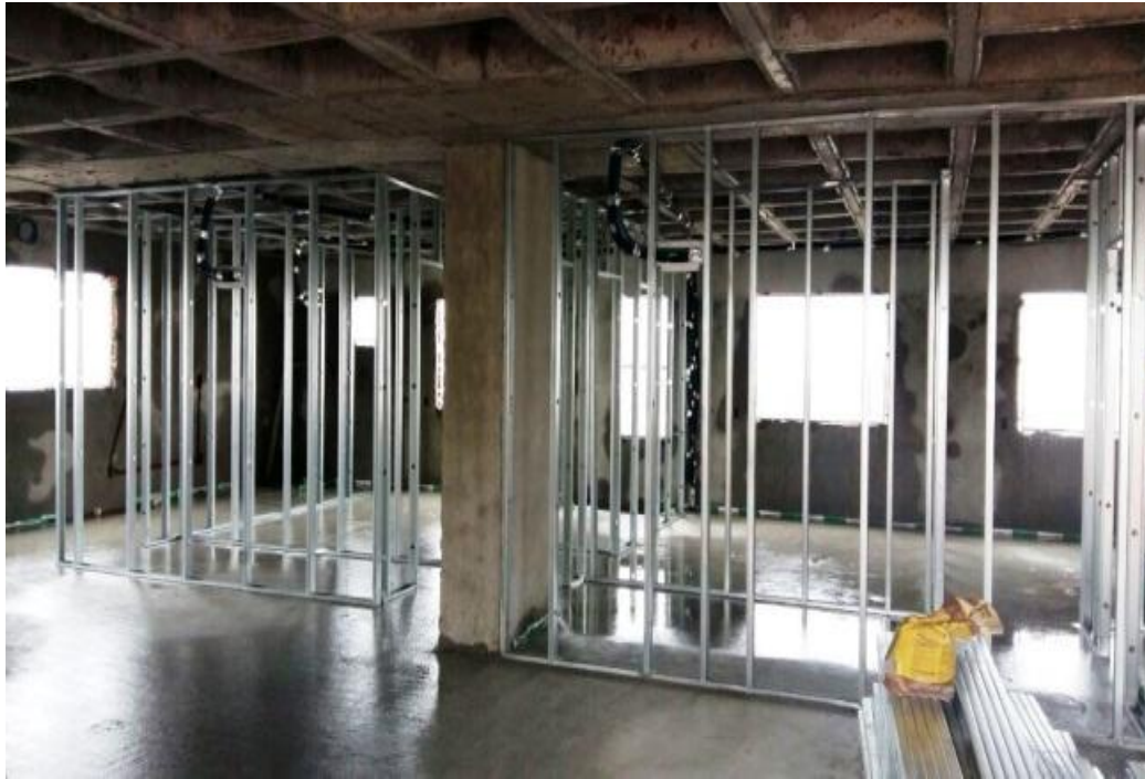
Fig. 6: Arrangement of the plaster in the apartment
