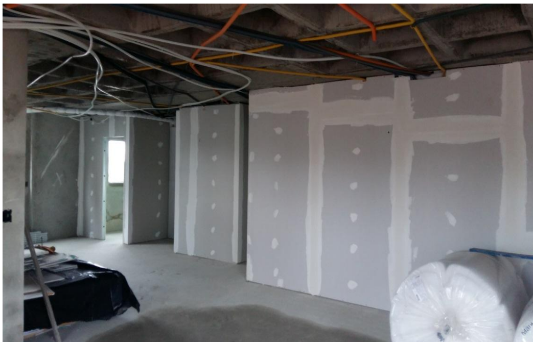
Fig. 7: Arrangement of the plaster in the apartment
