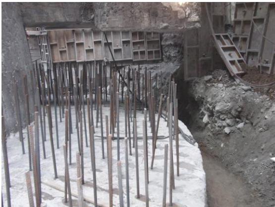
Fig. 6: Anchor works in chimney foundation
