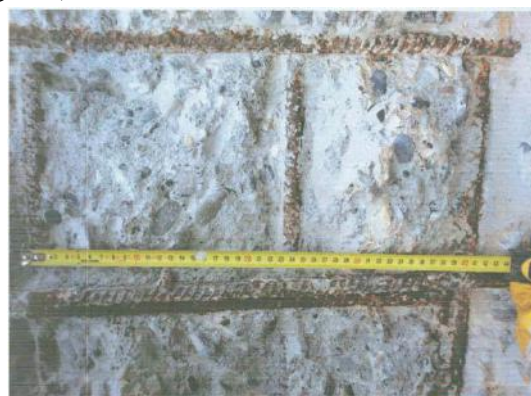
Fig. 3: Reinforced Steel Bar Pull Detection Activities
