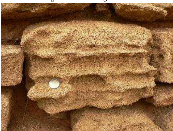
Fig. 7: formation, on the stone surface, of deep interconnected cavities
