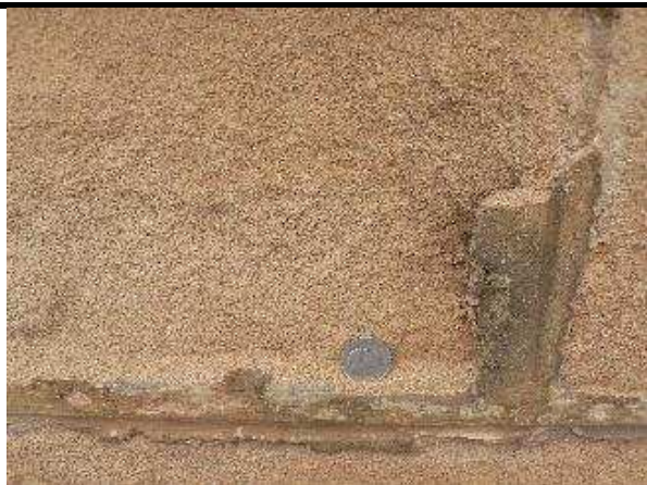
Fig. 6: Granular decomposition of a block of calcarenite, consequence of the use of a hard cement mortar. The rock has grown into a single alveolus.
