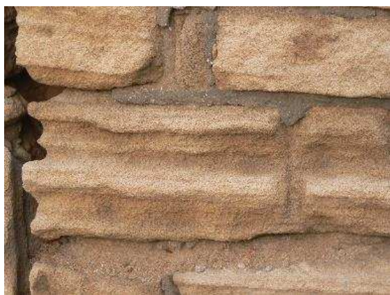
Fig.8: In contact with cement mortar, the rock has deep grooves that hollow out the material highlighting the hardest levels
