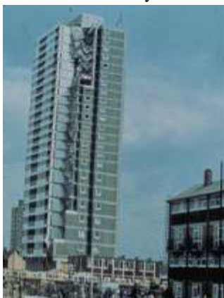
Fig.7: Progressive Collapse Ronan Point, UK, 1968[3]
