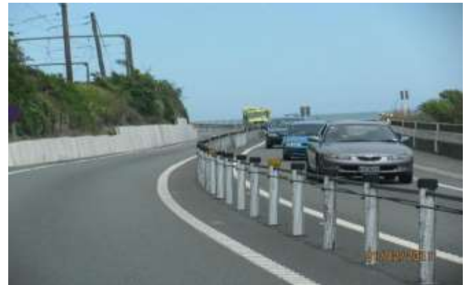
Fig.3: Flexible cable barriers
