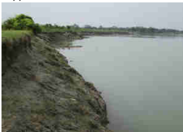
Fig.2: View of riverbank erosion at Neulgaon
