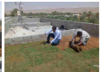
Figure: (12) Shows installation of final layer grass rolls (Bermuda 419 or Tifway).
