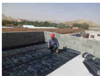
Figure: (7) Shows installation of (SBR) waterproofing membrane on 14-3-2014.
