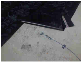
Figure: (14) Shows the installation of thermocouples sensors in substrate.
