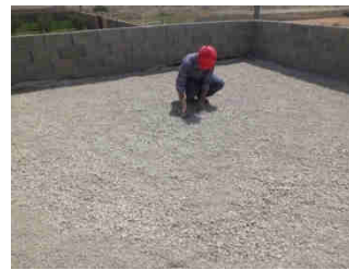
Figure: (9) Shows gravels layer 3cm (drainage layer) on 14-3-2014.
