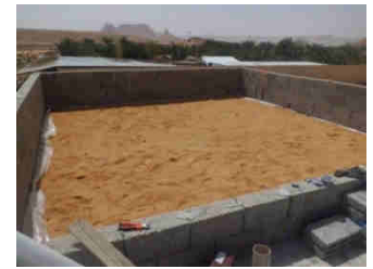
Figure: (10) Shows sand layer (drainage layer) 2cm on 14-3-2014.
