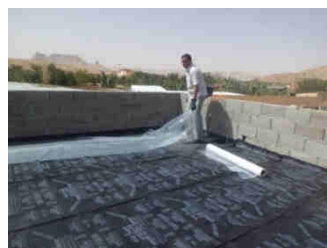
Figure: (8) Shows installation of polyethylene slip sheet on 14-3-2014.
