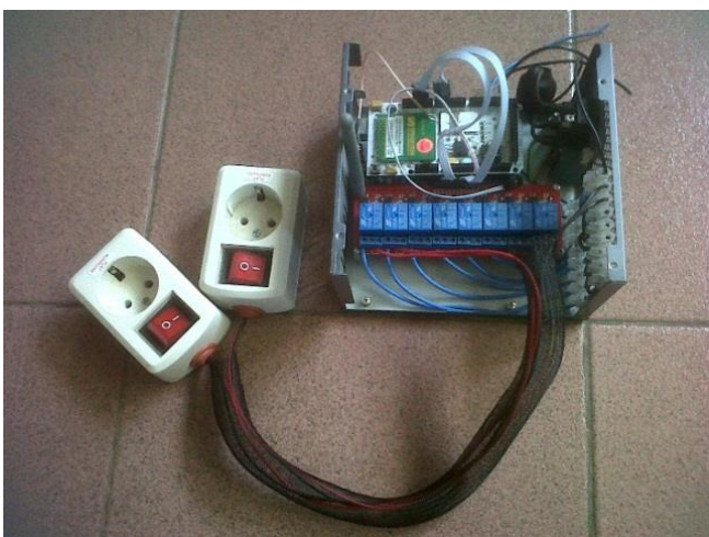
Fig. 5 Implementation of The Tool is Connected to The Electrical Terminals
