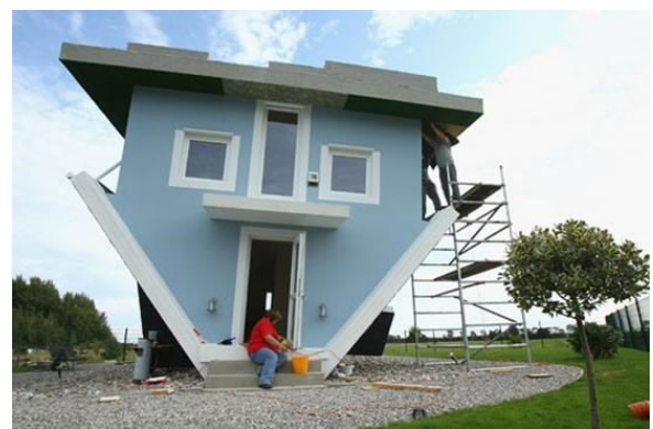
Citra 2. Proses Konstruksi The Other Upside Down House di Jerman
