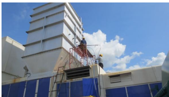
Figure 4. Installing sampling holes
