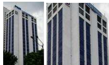
Gambar 8. Sirip-sirip semipermanen Wisma Arthaloqa Sumber: Survey, 2009
