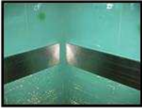
Gambar 21. Handle lift RS. Moewardi Sumber: Survey Lapangan, 2009
