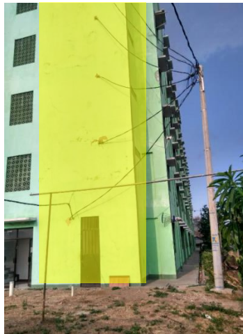
Gambar 3.8 Tampak Samping Kiri Rusunawa Kodam III/Siliwangi Jl. Tongkeng
