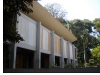
Gambar 4.13 Warna Dinding Masjid Salman ITB
