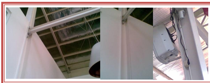
Gambar 3.4 Dinding Brussels Springs Resto and Café (Sumber: Dokumentasi Pribadi)
