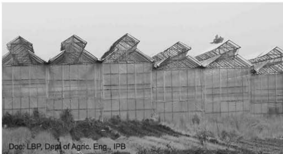
Figure 1. A multi-span piggy back structure with polyethylene film cover
