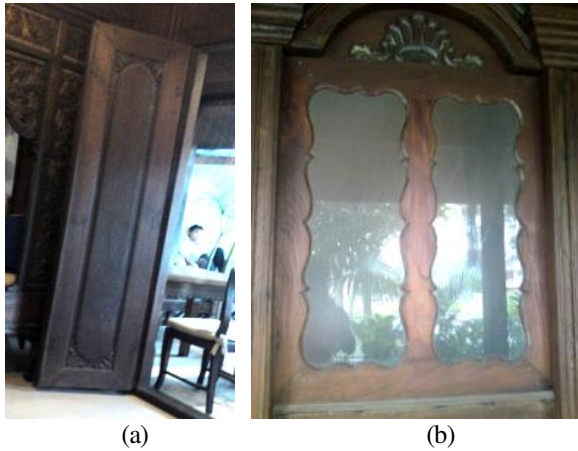
Gambar 7. (a) Pintu Nirwana Hall (b) jendela Nirwana Hall
