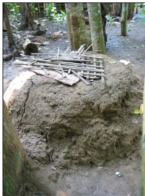
Pit latrine in flooding-prone area
