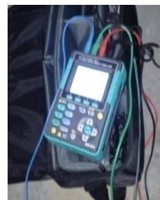
Gambar1. Power Quality Analyzer
