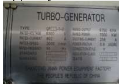
Gambar 2.9 Generator PLTU Biomassa PT. Suka Jaya Makmur
