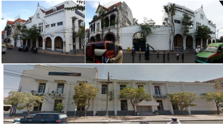
Fig. 11. Mandiri Building. (Researcher, 2016 and Google Earth )
